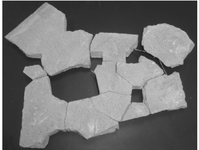
Fig. 7. Deteriorated panel that was broken apart in order to test the concrete and glass, 2009. Steel reinforcement made it difficult to separate the concrete fragments.
