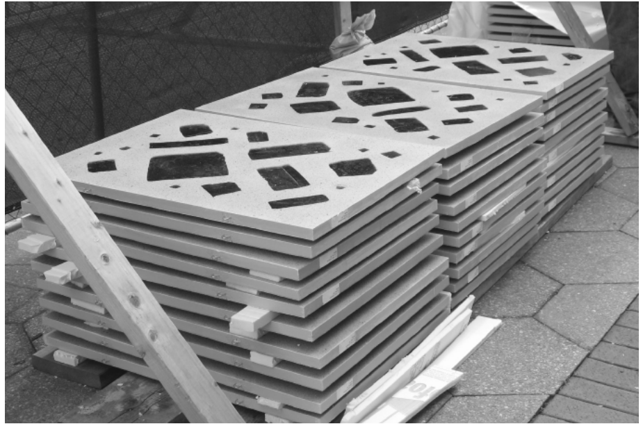
Fig. 11. New replacement dalle-de-verre panels with an epoxy matrix matching the exterior appearance of the original pre-cast concrete panels, 2009.
